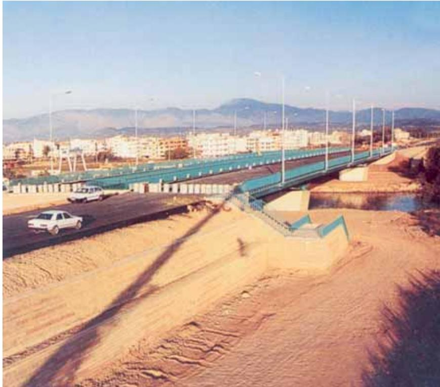
*Manavgat Bridge is the first application in Turkey such that orthotropic slab segments have been used in a relatively short steel bridge has been constructed by means of variable slab height, and cantilever proceeding.*
