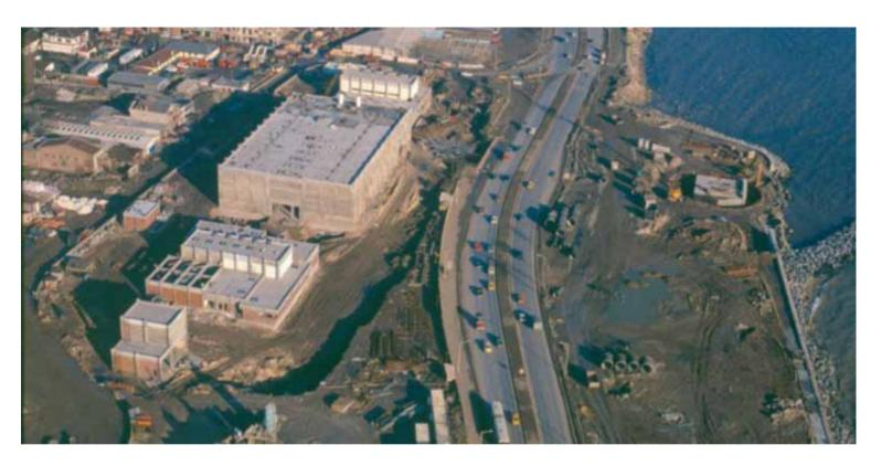
The pretreatment plant and outfall were designed for a maximum flow of 12 m³/s, some 1.6 times the average daily flows. The pretreatment plant to be located at Yenikapı, about 100 m. from the coast will include screening, influent pumping, aerated grit chambers, a grease removal channel and effluent pumping of flows larger than about 5 m/s.
