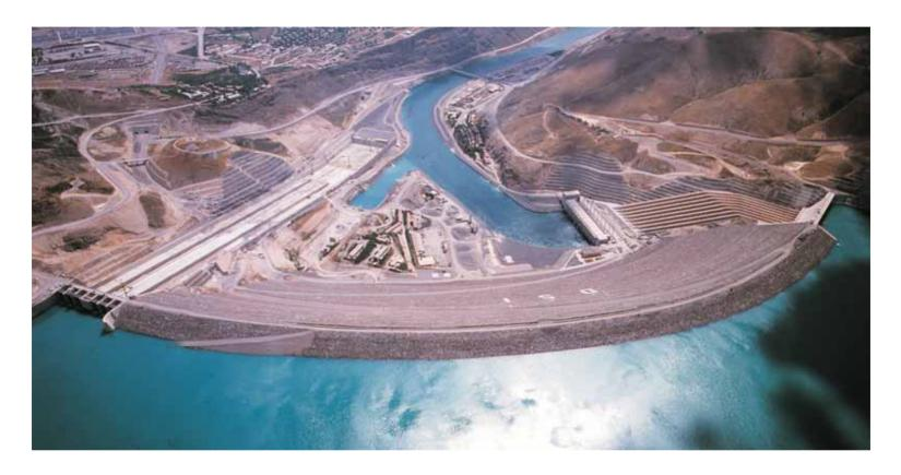
The Atatürk Dam is the largest in a series of 22 dams and 19 hyroelectric stations built on the Euphrates and Tigris rivers in the 1980s and '90s in order to provide irrigation water and hydroelectricity to arid southeastern Turkey. Completed in 1993, the Atatürk Dam is one of the world's largest earth-and-rock fill dams, with an embankment 184 m high and 1,820 m long. Water impounded by the dam is fed to power-generating units at Şanlıurfa that have a capacity of 2,400 MW.
