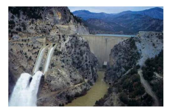
The dam has two spillway tunnels on the right side and has an underground power plant, installed power of which is 540 MW. Oymapınar Dam is nearly ten times greater than Seyhanlı Dam, five times than İrfanlı Dam and two times than Gökçekaya Dam in terms of electricity generation. In the construction of dam structure concrete has been used as filling material. Height of the dam is 185 m from the foundation and its length is 360
