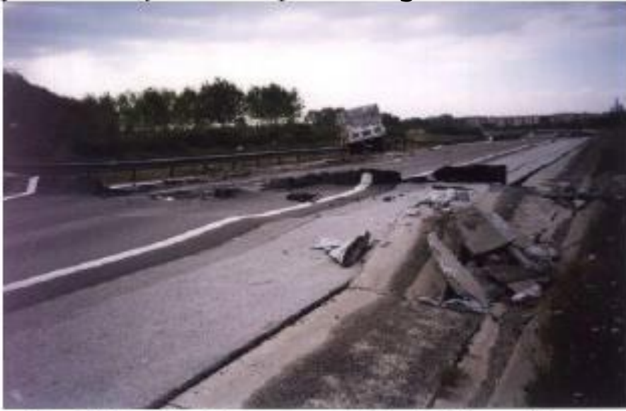
Figure 7.35: Buckling of the motorway surfacing (asphalt) near Arifiye
