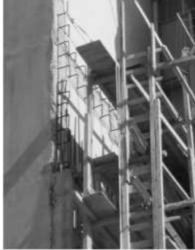
Figure D.6: Production of eccentric reinforced concrete shear walls.
