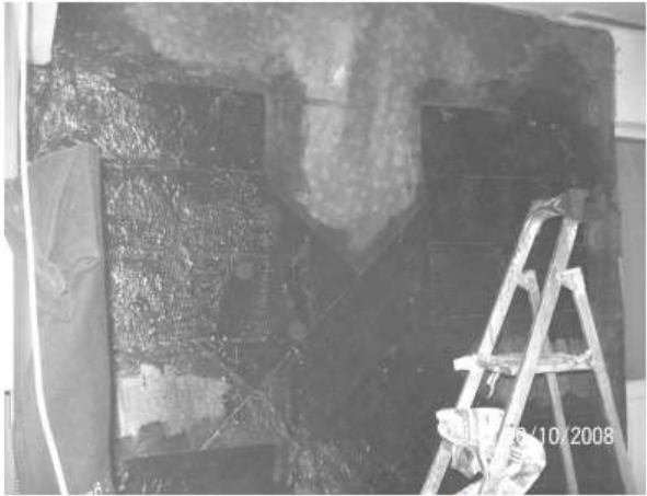
Figure D.3: CFRP Application on the masonry infill wall.
