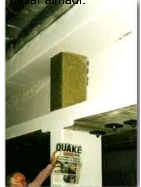
Figure 7. Retrofitted column at Hotel Nikko
