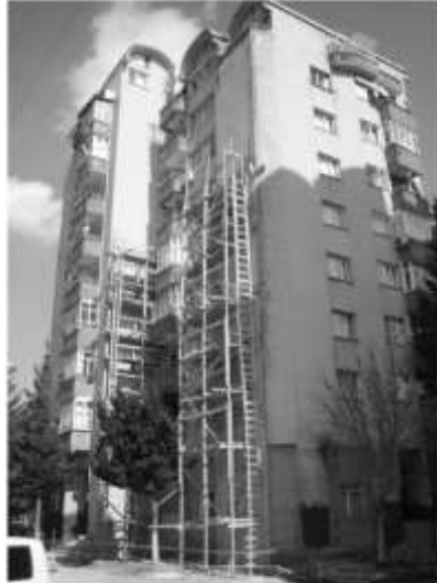
Figure D.7: Production of eccentric reinforced concrete shear walls.
