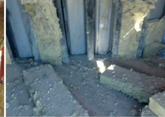
Failure of Interior Finishing Panels of Ground Unit
