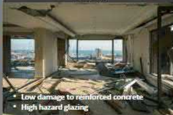
OBSERVED BUILDING DAMAGE (estimated distance from blast site)
