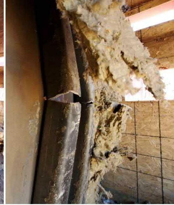
Ground Unit - Glazing Framing and Surrounding Damages
