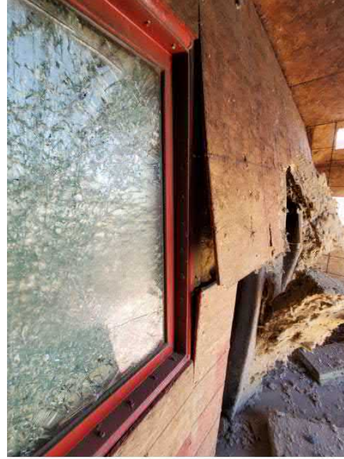
Ground Unit - Glazing Framing and Surrounding Damages
