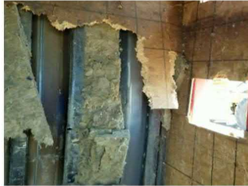
Failure of Interior Finishing Panels of Ground Unit
