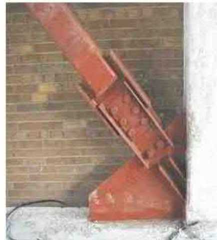
Friction damper in single diagonal bracing
