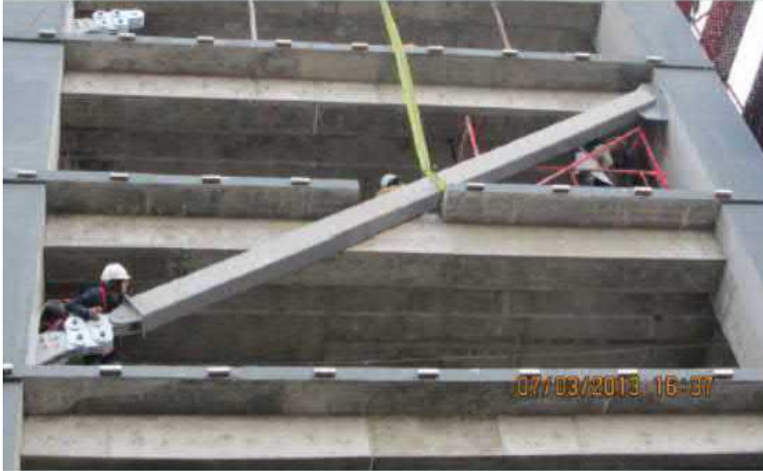
New Building in Chile 19 Floors with Diagonal Bracing
