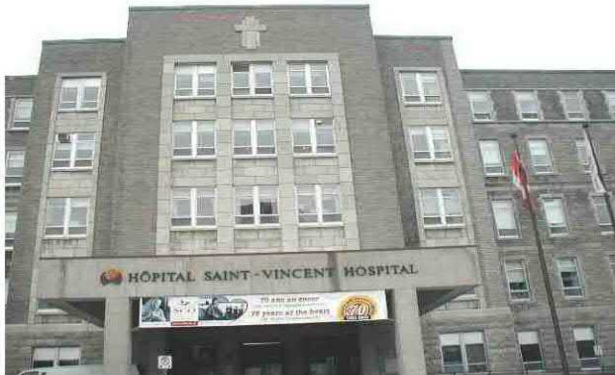
Figure 1, Front View of Wing-B (Partial)
