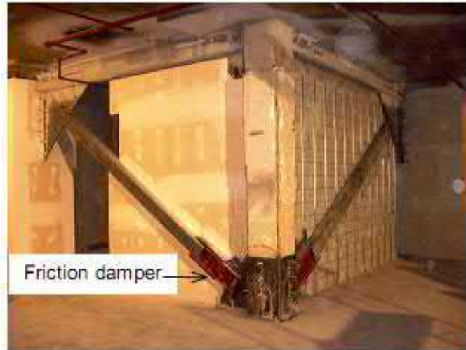
Figure 4. Friction damper in single diagonal brace.
