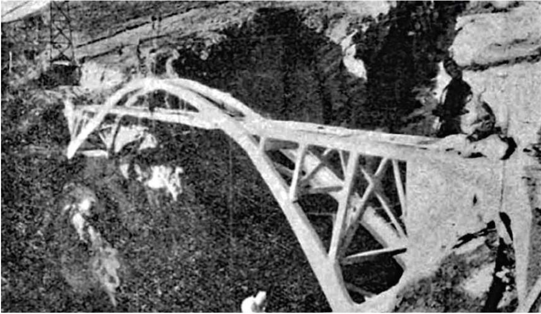
The bridge nearing completion, deck hangers and railing to finish "The novel feature of this bridge, apart from its great span (which is believed to be the greatest yet attempted in the British isles) and its height above the water, is that it was possible to erect without centering, thus effecting a great saving in cost." -Noel Ridley.
