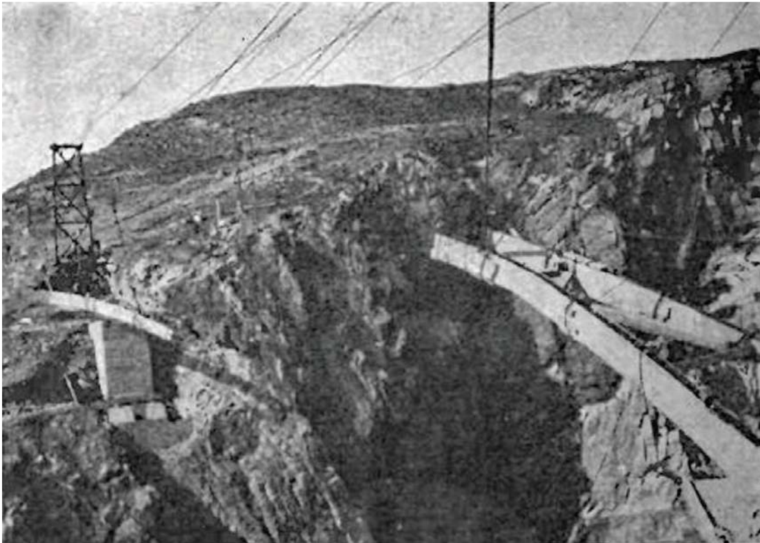
Winching the arch ribs troughs sections into position across the gorge. Part of the cable stay structure is seen on the left.
