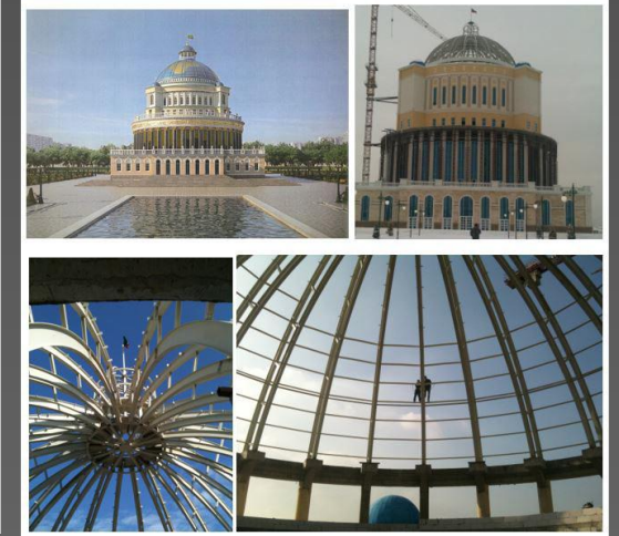
GROZNY OPERA HOUSE DOME 2009 RUSYA KUBBE ÇAPI 36 M (EUROCODE 3)
