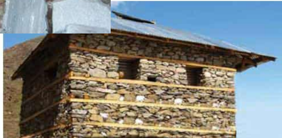
Contemporary Bhatar construction Tarand - NWFP - Pakistan
