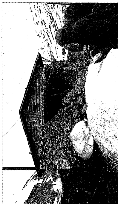
Figure 4 Partial Collapse of a Stone Masonry Building in the Mountain Village of Mecediyeh
