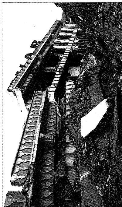
Figure 2 Bottom-up Collapse of RC Building in Karaağaç District, with Partial Survival of Upper Storeys
